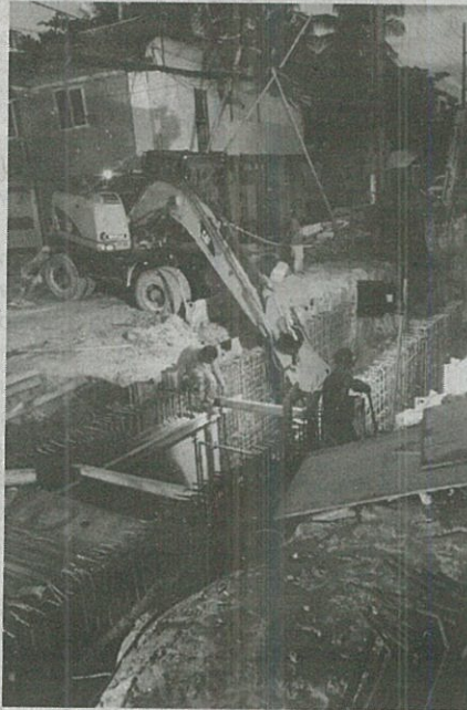
Left: Construction of an efficient drainage system. Right: Massive pipes were installed along Bolabog beach to improve the island's drainage system.
